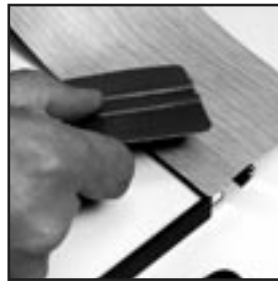
2. Burnish vinyl down around the header & base.
